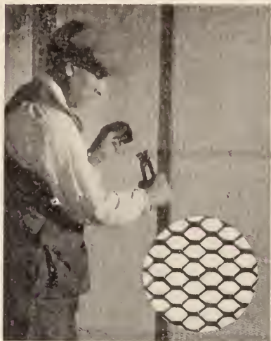
Myriads of tough steel strands strengthen the plaster against cracks.
